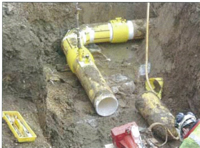
PE pipe being installed for gas distribution
