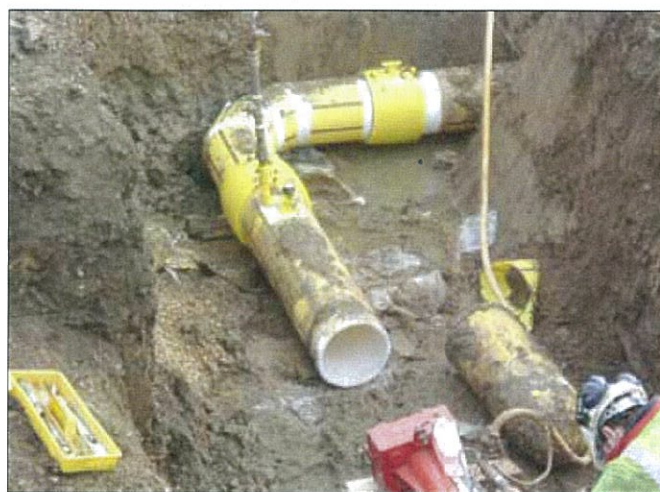
PE pipe being installed for gas distribution
