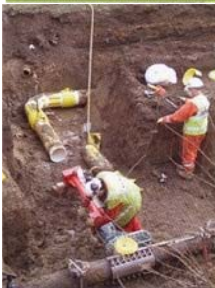
TYPICAL SITE CONDITIONS FOR INSTALLING PLASTIC PIPES
