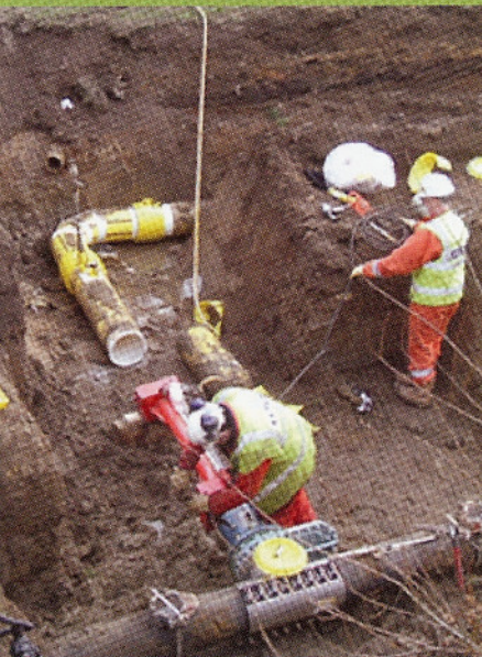
TYPICAL SITE CONDITIONS FOR INSTALLING PLASTIC PIPES.
