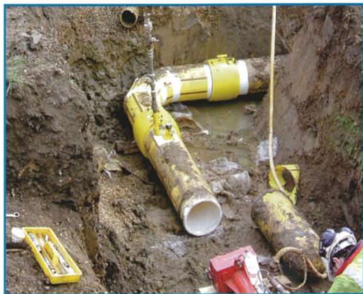
PE pipe being installed for gas distribution
